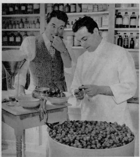
No cosmetics expert, Bradley watches Dick Bagley, head chemist, preparing foundation cream. First steps: Plucking stems, grinding berries, filtering. Liquid in jar is from a quart of berries. All work is done by hand
